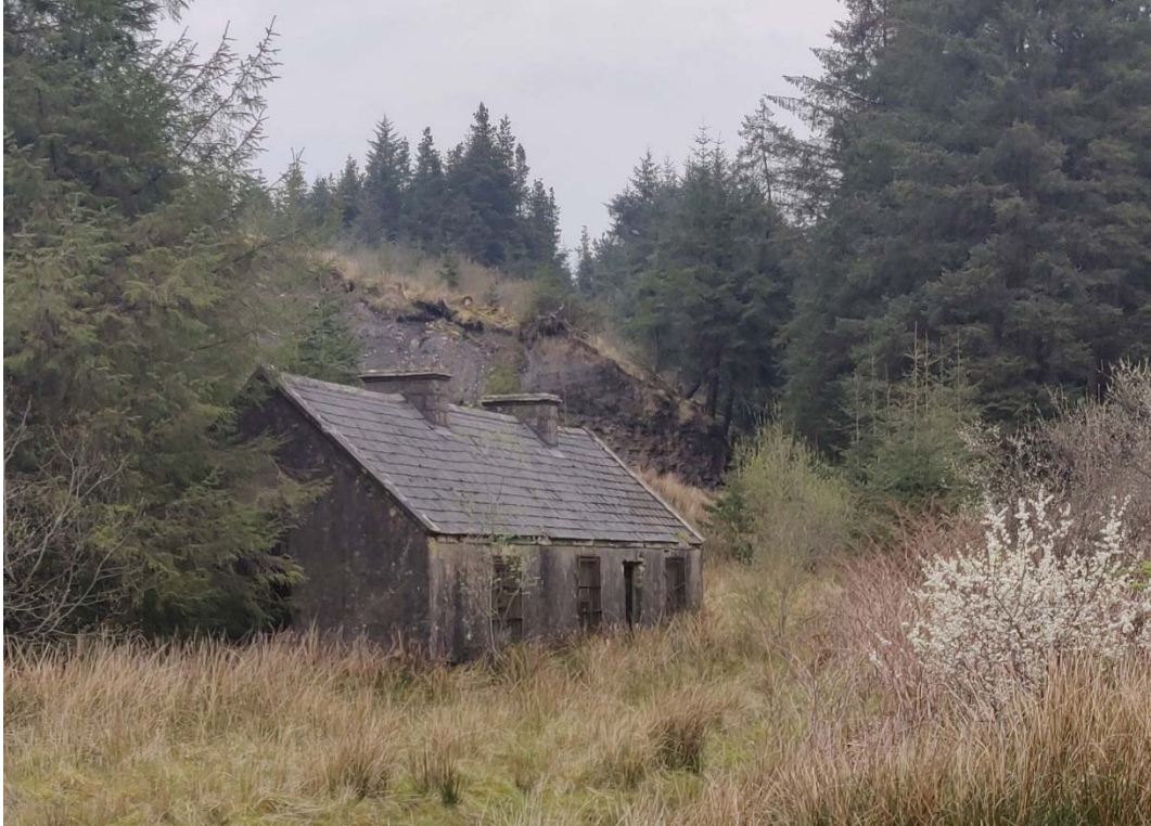
Plate 4.1 Derelict dwelling located on site.
